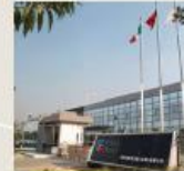
PRIMA POWER SUZHOU CO. LTD Suzhou, China
