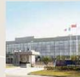
PRIMA POWER SUZHOU CO. LTD Suzhou, China
