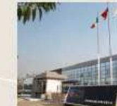
PRIMA POWER SUZHOU CO. LTD Suzhou, China
